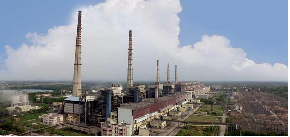
Picture: (Captive Power Plant | NALCO (National Aluminium Company Limited) | A Govt. of India Enterprise)
