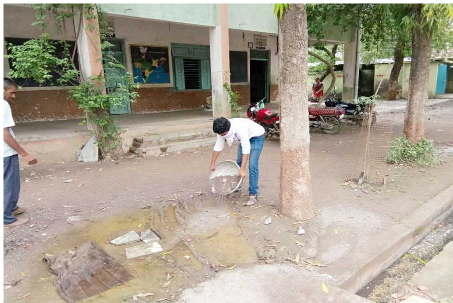
F) Cleaning the drainage by removing the solid waste.
